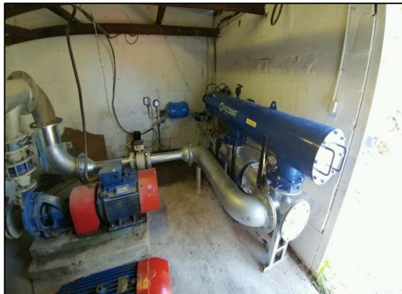
The new filter in the pump house
